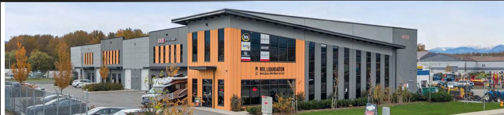
YALE ROAD BUSINESS PARK 44703 Yale Road, Chilliwack, B.C.
