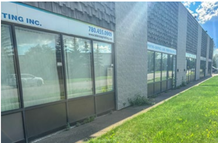
Masonry Construction with Updated Roof
