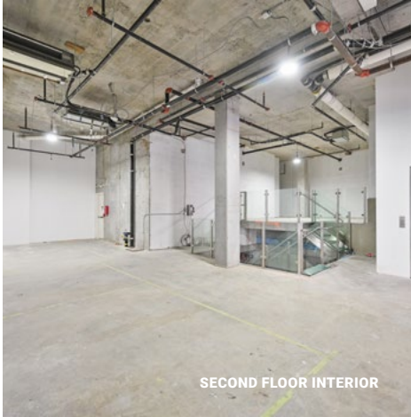
SECOND FLOOR INTERIOR
