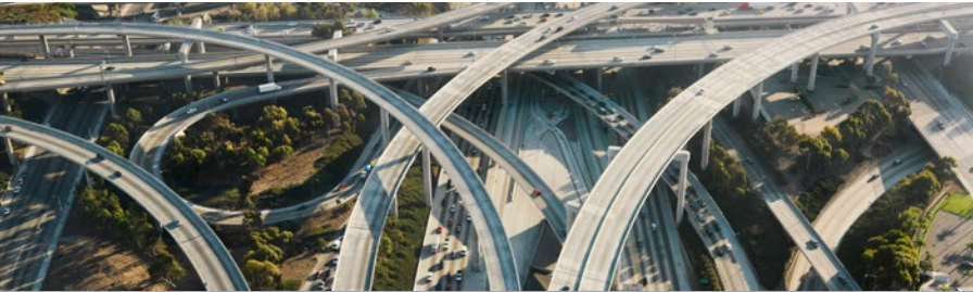
CLOSE PROXIMITY TO 400 SERIES HIGHWAYS
