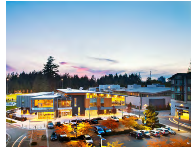
Wesbrook Village is home to the Wesbrook Community Centre and the University Hill Secondary School
