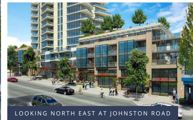
LOOKING EASTTOWARDS MAIN LOBBY ENTRY
