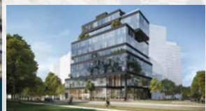
220 Prior Street 102,000 SF Office, industrial, retail
