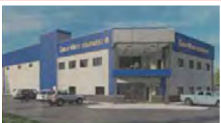
Great West Equipment 7411 Riggs Cr 40,000 SF Logistics Warehouse
