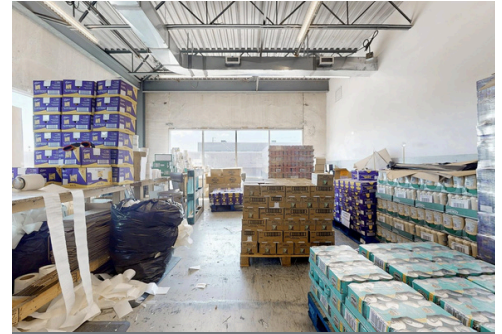
Upper Level Industrial Area
