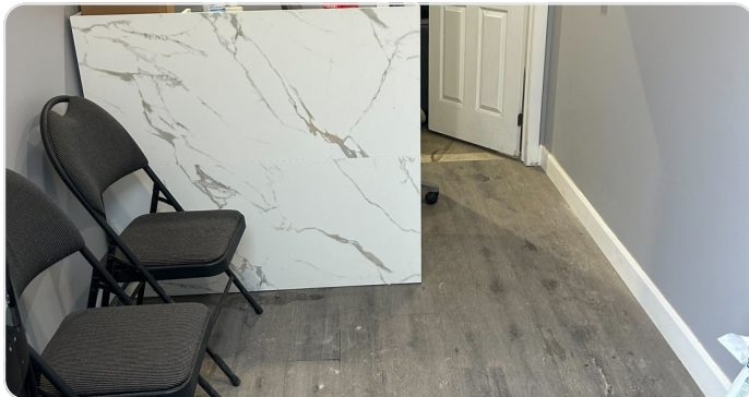
Finished front office and reception/waiting area, separated from the bay
