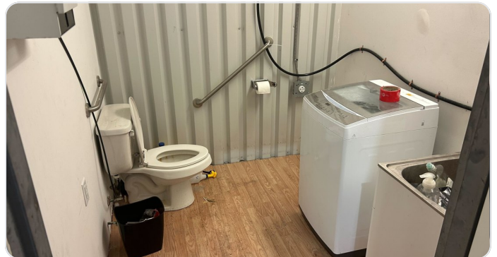
Full washroom with ample space for a washing machine and dryer
