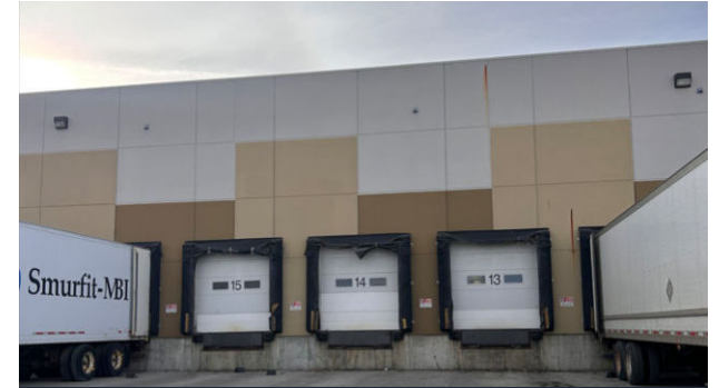
Cross Dock Exterior Loading
