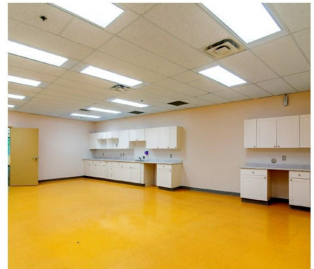
Testing / Lab Space with Plumbing
