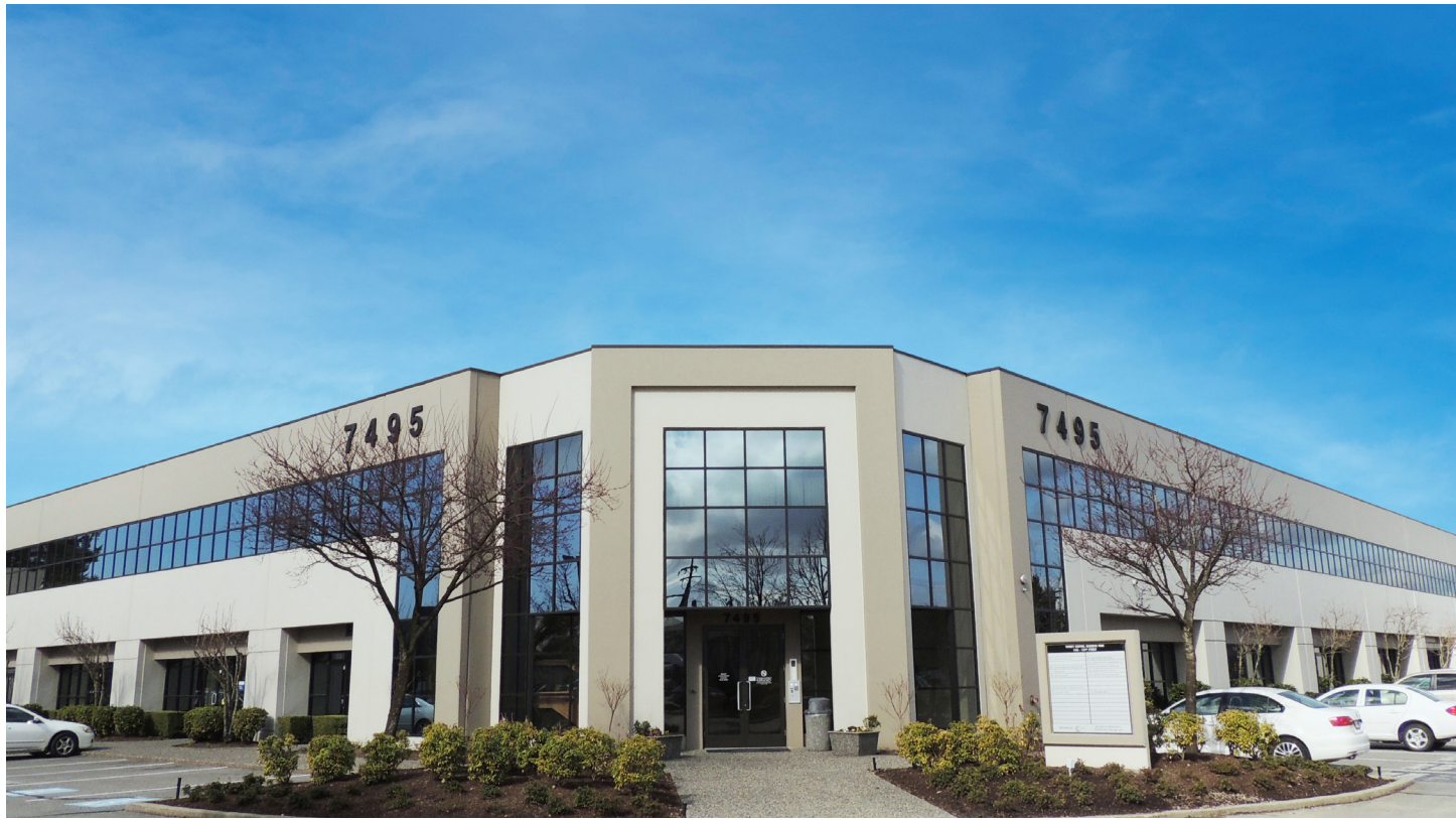
BUILDING 2, 7495 132ND STREET
