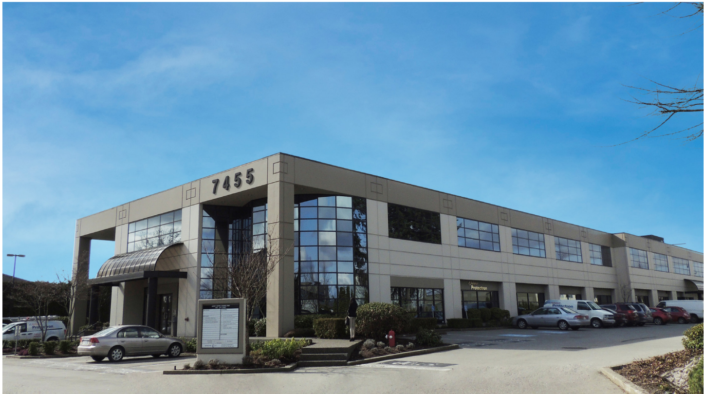
BUILDING 4, 7455 132ND STREET
