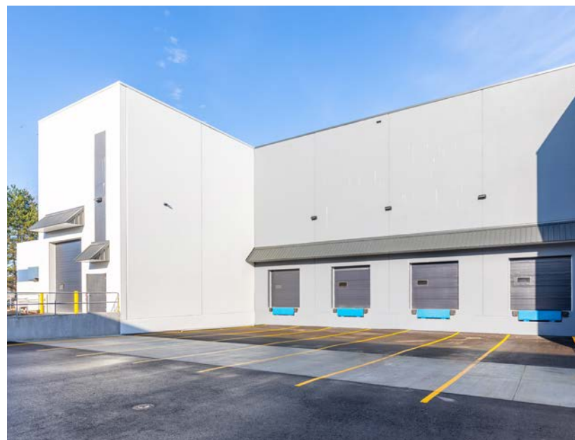
Roof Installation Completed June 2025
