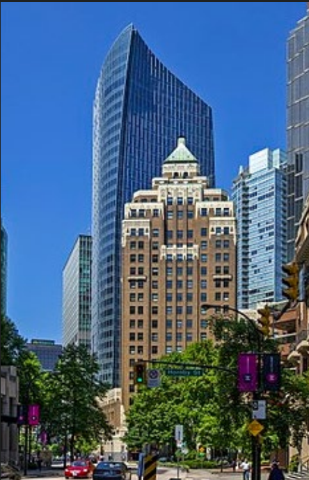
MNP TOWER VANCOUVER, BC
