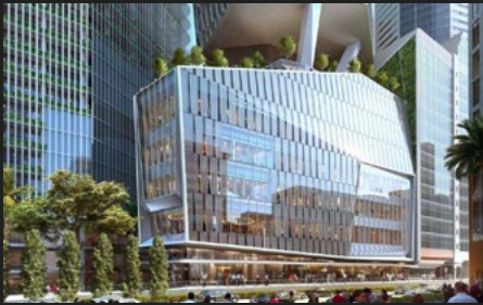
ROBINSON TOWER SINGAPORE
