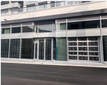
Exterior Street Frontage
