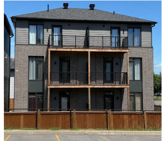
East Block – 4 Unit Building
