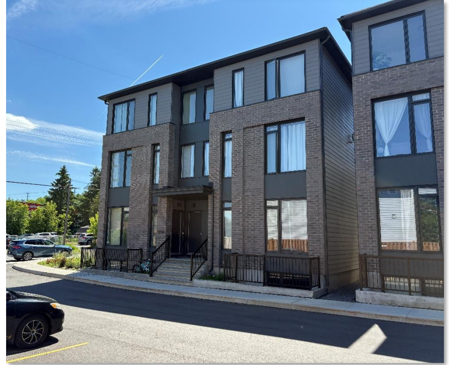
East Block - 4 Unit Building
