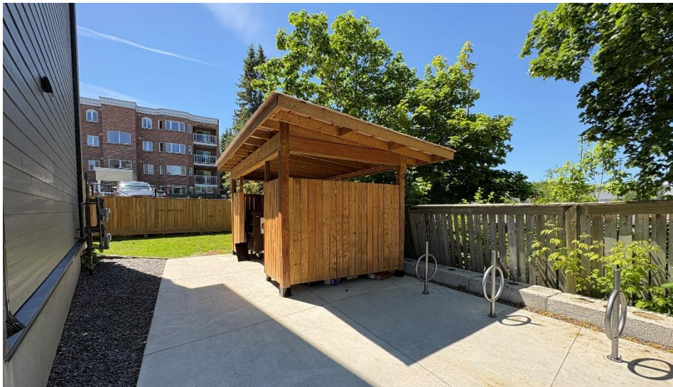
Garbage Structure & Bicycle Storage
