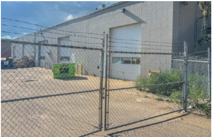
Fully Fenced & Gated | 17' Clear Ceiling Height
