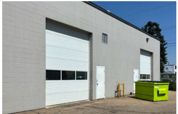
Paved Yard with Catch Basin
