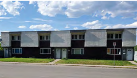
PARKCREST COURT | 46 UNITS 1520 & 1602 1st Street, Cranbrook, BC
