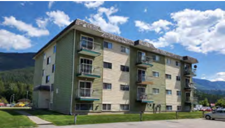
PINEWAY COURT | 46 UNITS 525–575 Pine Avenue, Sparwood, BC
