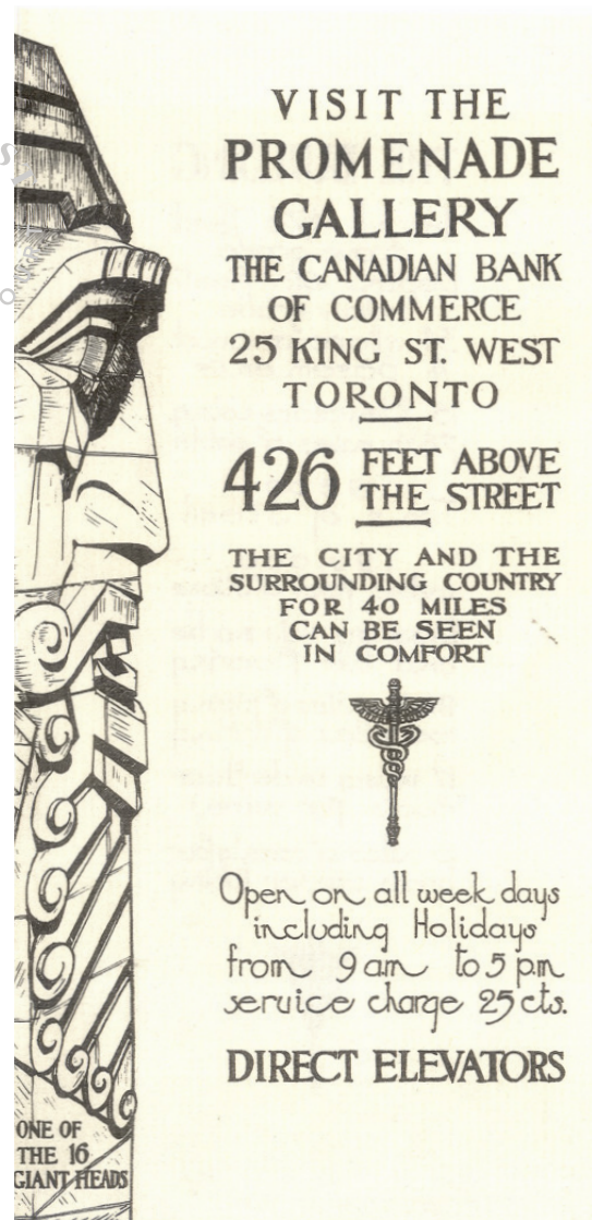
As the tallest building in the British Empire and Toronto's first "skyscraper," the North Tower drew crowds to its 32nd floor Observation Gallery.
