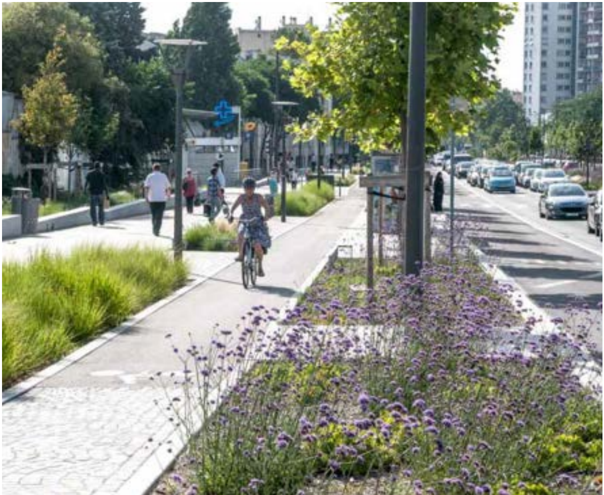
Complete street design with wide sidewalk, separated bike lane, stormwater facilities, street trees, and on-street parking
