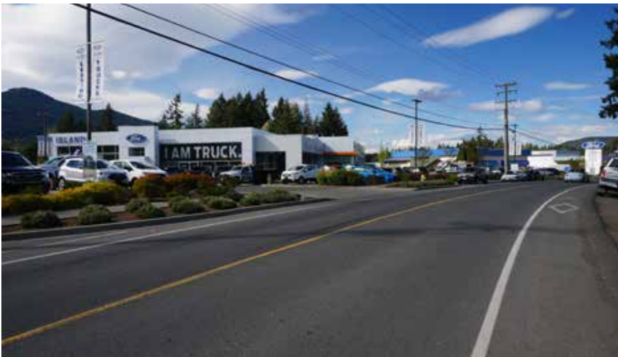
Despite road improvement in some locations, on-site pedestrian and cycling facilities are largely absent in the area
