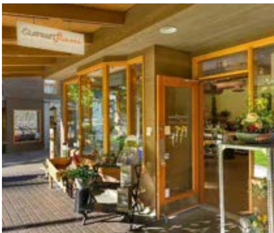
High quality build materials and architecture
