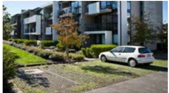
Permeable paving in a surface parking lot
