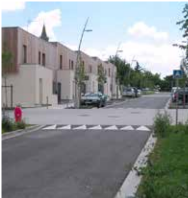
A raised pedestrian crossing
