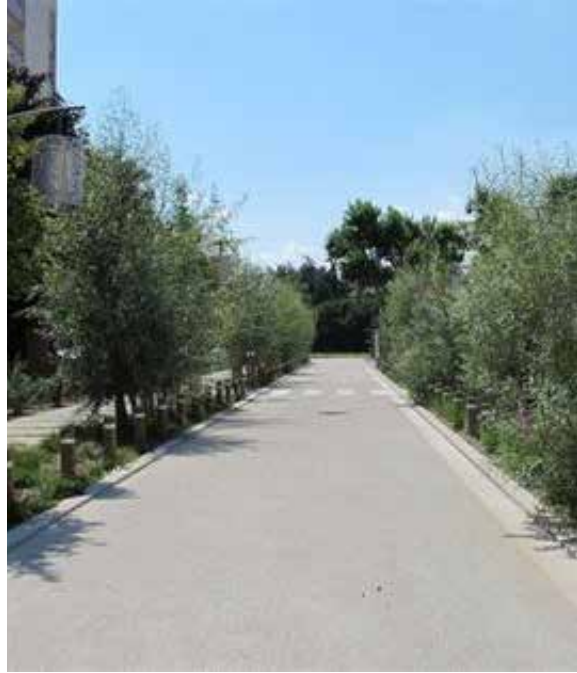
Shared space street with multi-functional landscaping
