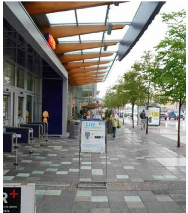
Building overhang providing weather protection
