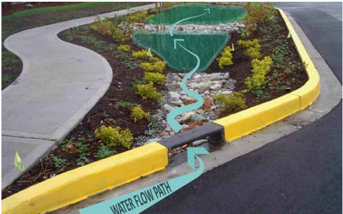
Stormwater flow path into on-street raingarden
