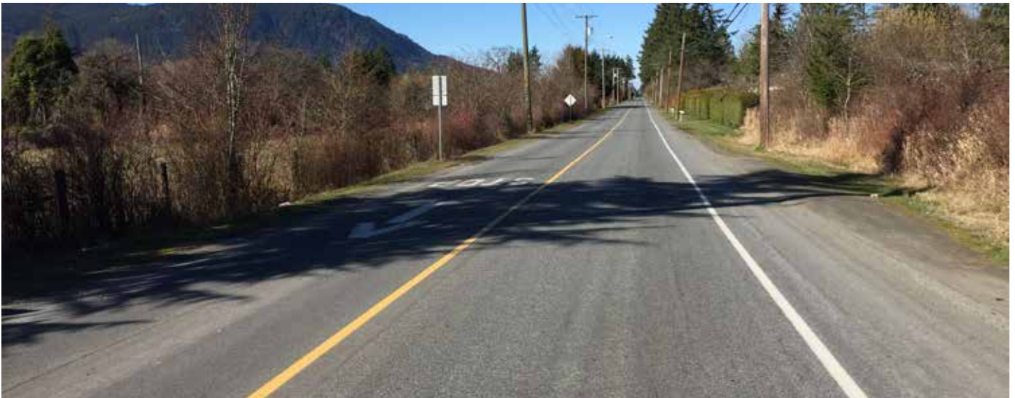
Bell McKinnon Road, today, with no pedestrian or cycling facilities
