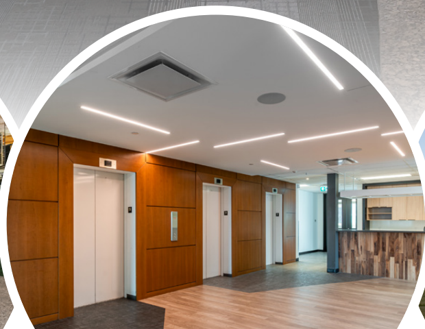
UPGRADED ENERGY EFFICIENT ELEVATOR SYSTEM
