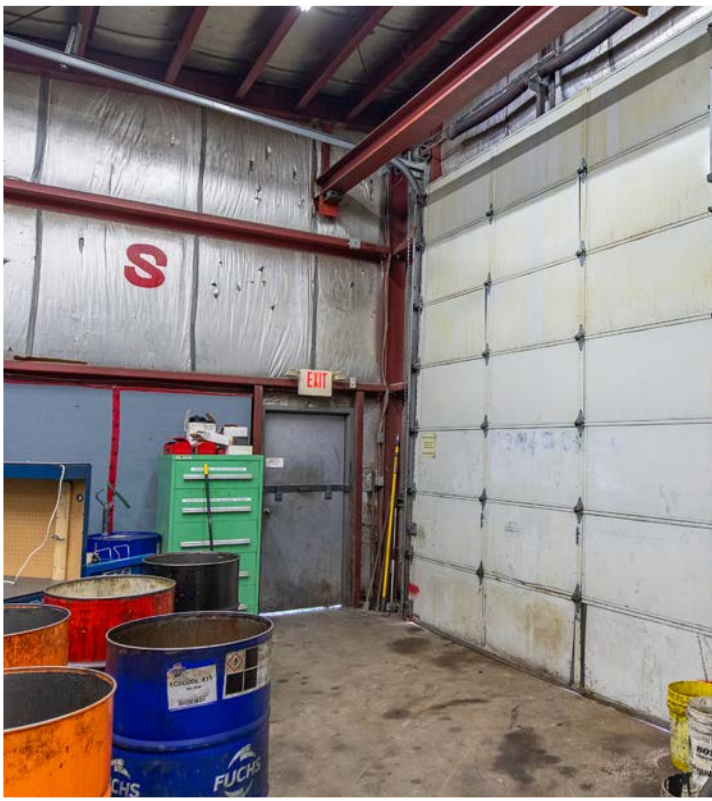
Interior Building Photos
